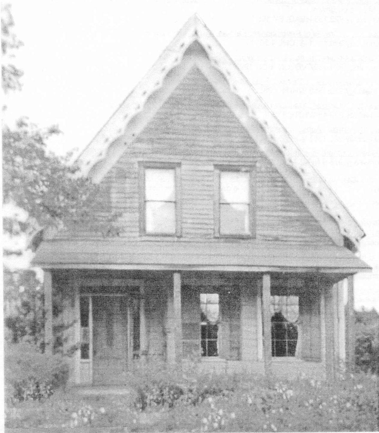
Crosby House c1950 as found by Daughters of the Pioneers (Photo credit: Daughters of the Pioneers - Crosby House Collection). See the cover for the Crosby House as it appears today.
